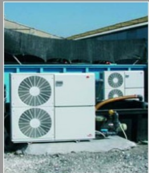
Fig 82 - Heat pumps
