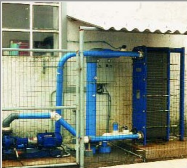
Fig. 81 - Heat exchanger
